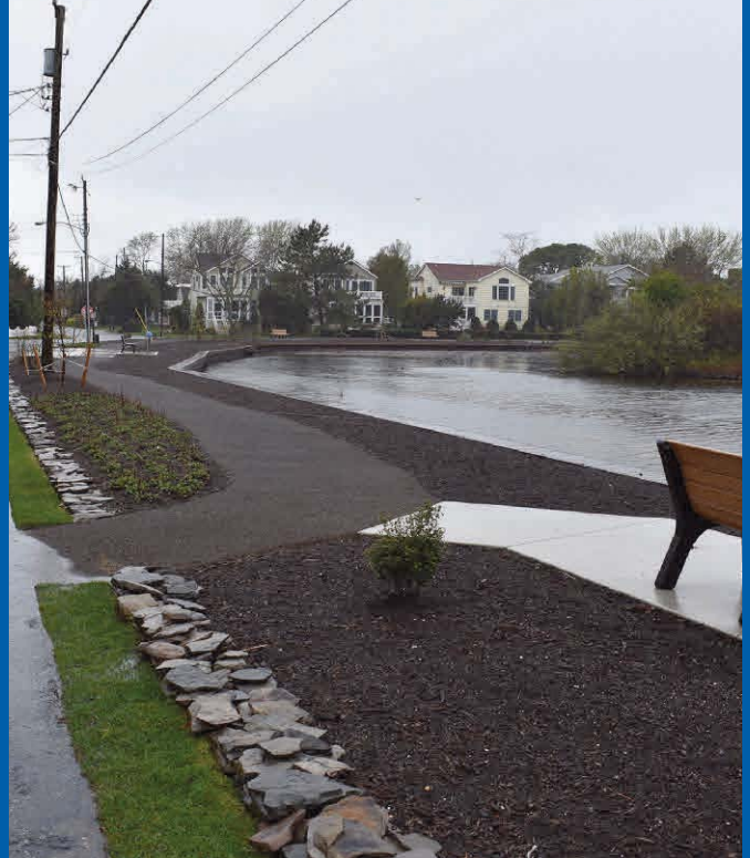
West Bay installed a meandering porous walkway along the park banks of Lake Lily in Cape May Point
