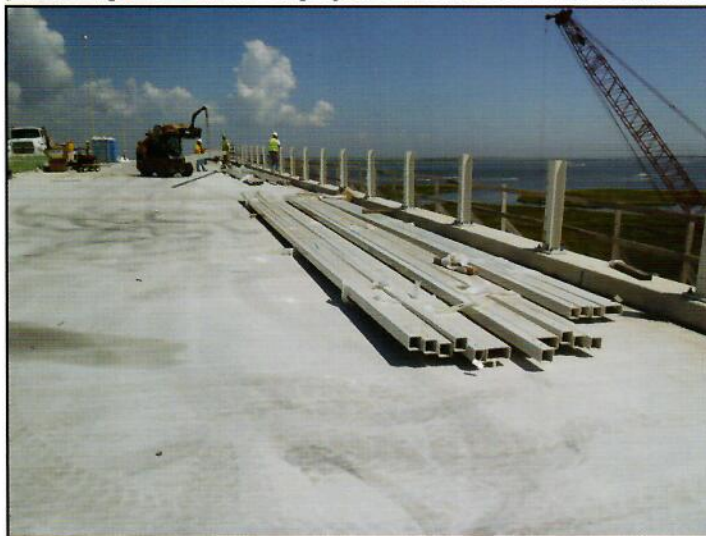
West Bay installs bridge and pedestrian rails on the Route 52 project.
