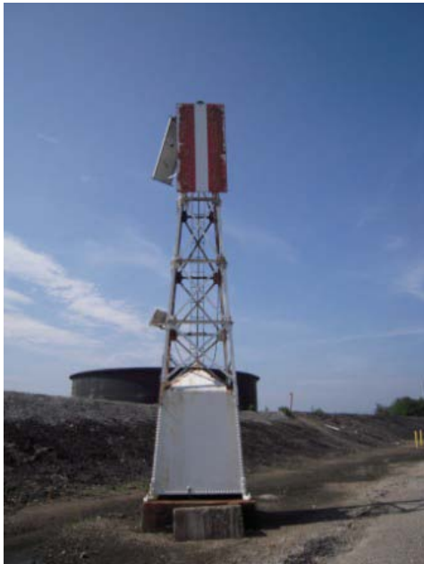
Rear Range Tower - Before
