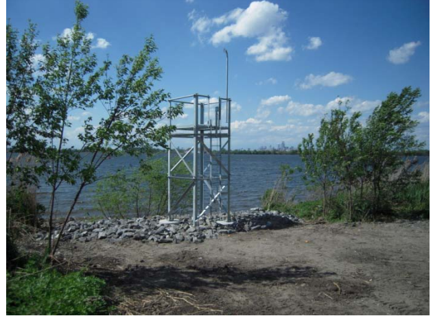
Front Range Tower - After
