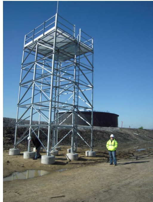
Rear Range Tower - After
